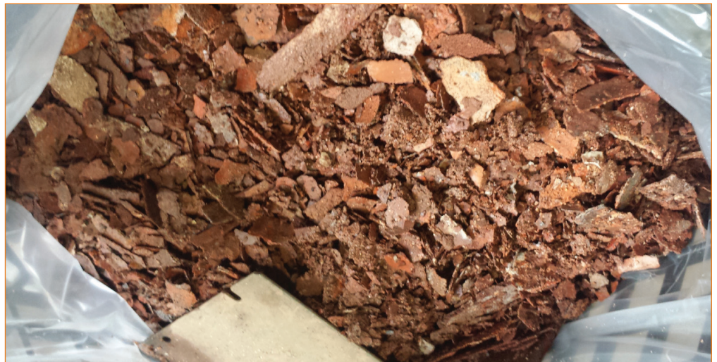
This scale buildup was manually removed from a water system.
